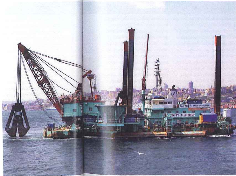
Istanbul has a remarkable list of infrastructure projects, like the Marmaray rail tunnel beneath the Bosphorus river.
